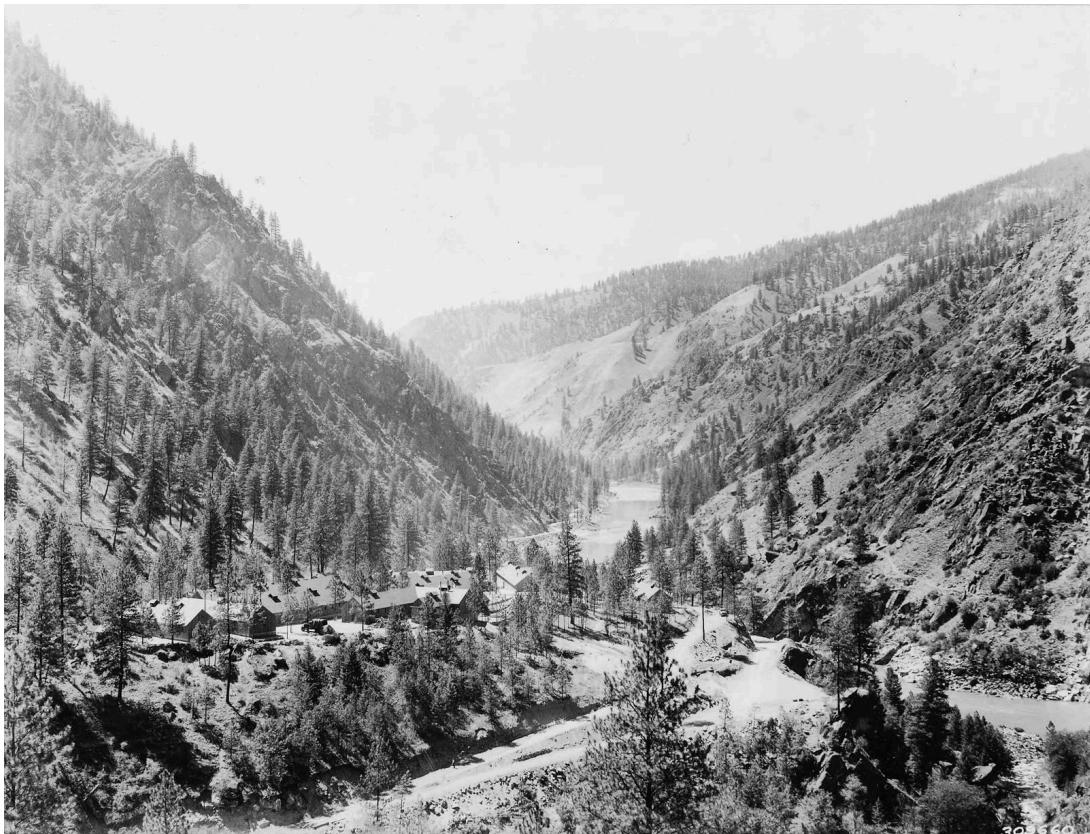
CCC Barracks at today's Salmon River High Adventure Base - https://www.lib.uidaho.edu/digital/cccidaho/items/cccidaho110.html
